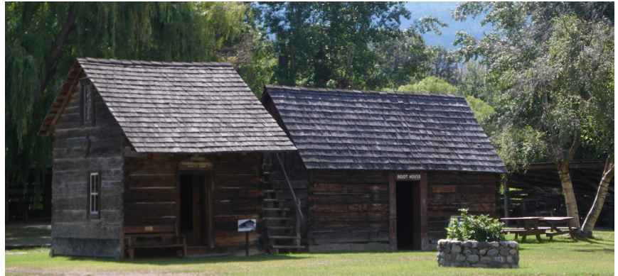
The restored chapel (on left) and root house (on right) at the Mission of the Immaculate Conception aka Father Pandosy Mission. The sign in front of the chapel says, "The Immaculate Conception Mission Chapel was the first original two story building constructed in 1860. The building was constructed by Brother Surel OMI, the carpenter of the group, along with Father Pandosy OMI and Father Richard OMI. The lower floor was used as a Chapel while the upstairs was used as a school and living quarters for the priests." Photo Credit: Carolin Robertson 25 July 2014.
