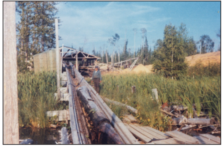
Jackladder at Crawford sawmill, Otto Lake (west of McCullough Lake) late 1960s
