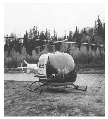
Waterlogged - Bob Stevenson sends this photo of pilot Frank Arman and a Bell 47J-2 near the confluence of Wabasca and Muddy rivers, 1966. He writes: "The machine refused to start after we endured a 'micro-burst' shower, forcing us to check and dry the wiring harness and plugs before it would fly. The J-2 was our vehicle for a tree growth and spruce budworm project in the Wabasca area."
